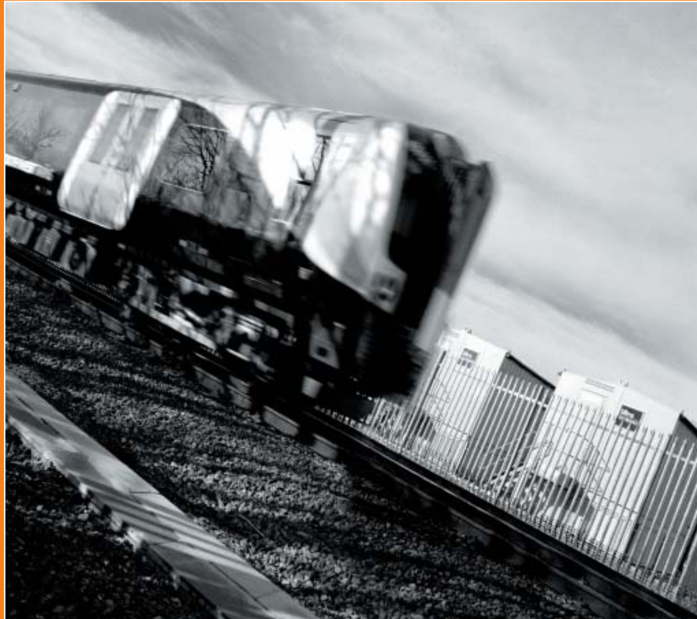
Ultra's power equipment for Southern Region
